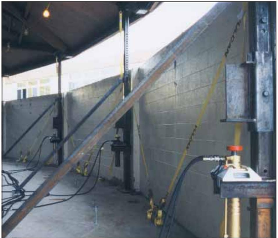
ASM System jacking posts lifting dome 4'1".
