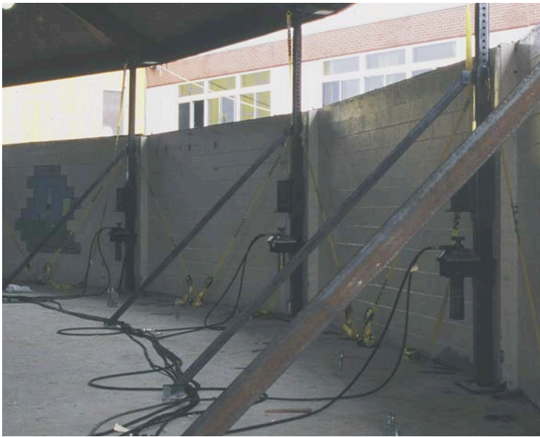
Hendrick Hudson High School jacking posts set in place
